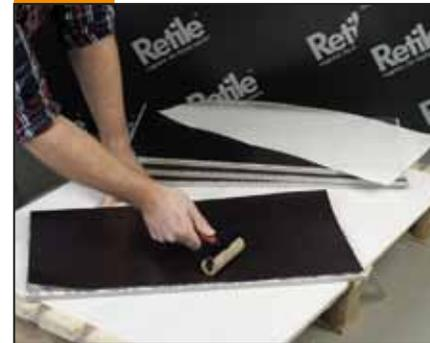
Position the Retile Magnetic Panel over the tile back and apply pressure with the Retile Application Roller to ensure a solid bond.
