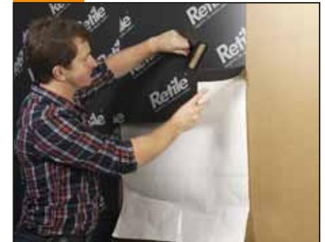
Peel back the release liner a little and start to apply to the sealed substrate. Use the Retile Application Roller to apply pressure to the panel, ensuring no air bulbs.
