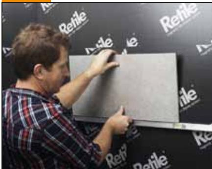
Using the Retile Spirit Level as a stop, place your magnetised tile on to the wall and away you go.
