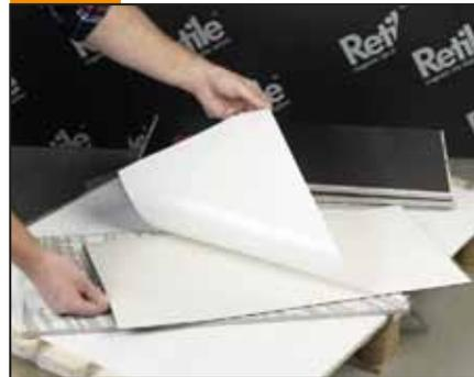
The Retile Magnetic Panels are supplied pre-cut to your specified size. Peel back the release liner to expose the special high bond adhesive.
