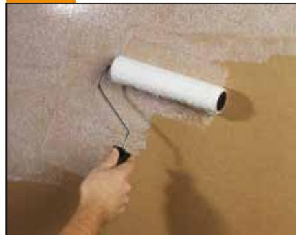
Start with a clean, flat substrate and seal it with a suitable primer and leave to dry.
