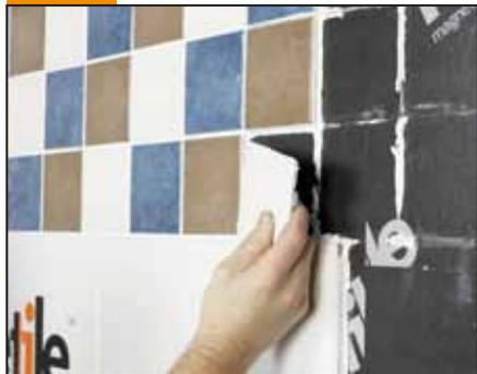
When you decide to refresh your displays, the tiles can be removed easily and once the wall is cleared of old grout, then the next tiles can go up.
